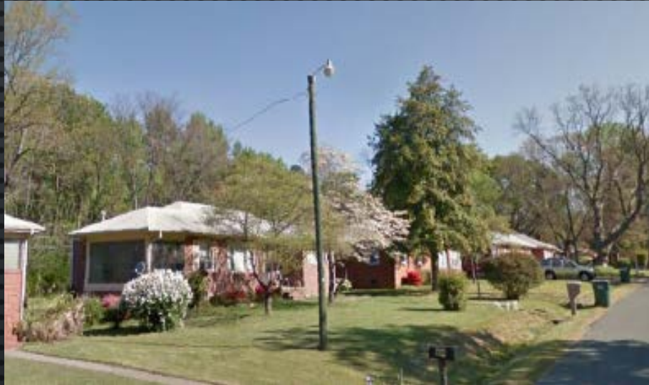
Standard Street Light on Wood Pole (Typical of 5000 Lumen HPSV)
