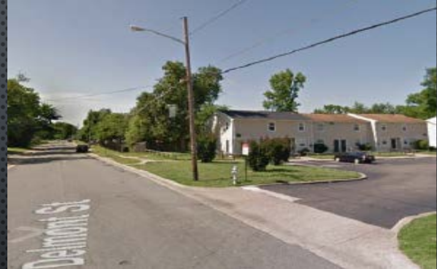
Standard Street Light on Wood Pole (Typical of 8,000 and 14,000 Lumen HPSV, Shown With 6' Arm)
